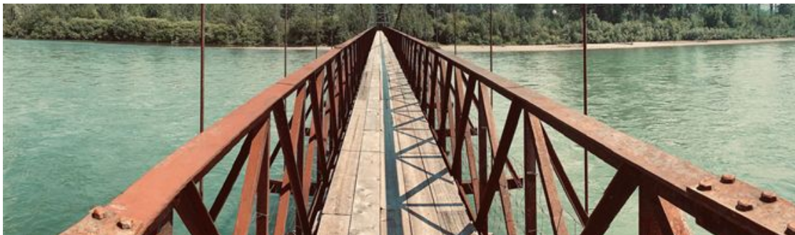
Photo credit: Kate Ames, Bulkley River Suspension Bridge.
