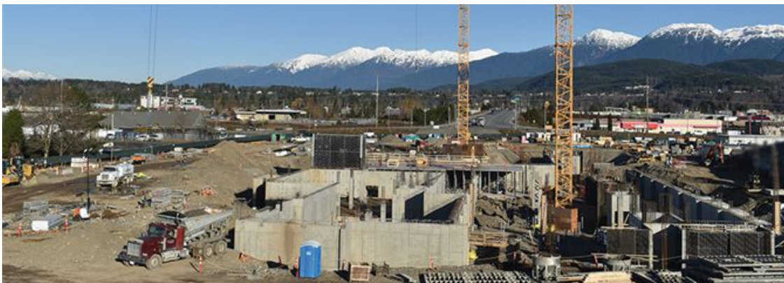
Mills Memorial Hospital Replacement project.
