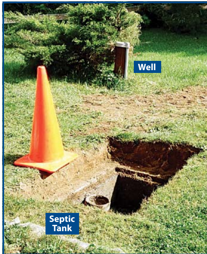
Figure 7. Well too close to septic tank – well/tank should be at least 15 metres (50 feet) apart
