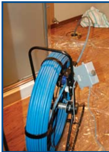
Figure 3. Using a pipe camera to find septic tank
