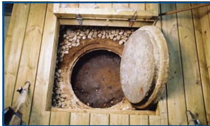
Figure 8. Exposed hatch in deck provides access to secure concrete tank lid
