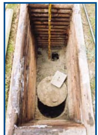
Figure 6. Deep septic tank in confined place – WorkSafeBC rules apply
